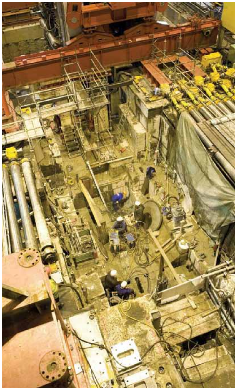
Roll Mill replacement project—BWW.
