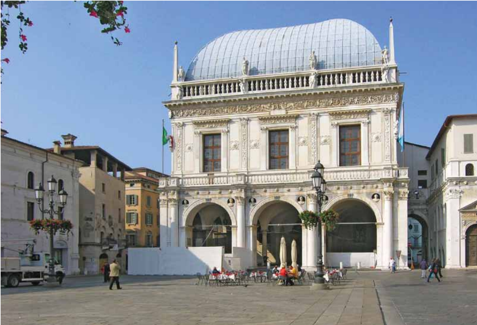
Loggia Palace foundation consolidation project—Tondin srl.
