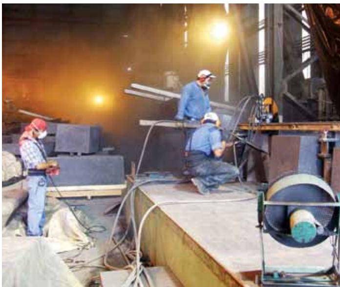
Crucible repair project—ADRA.
