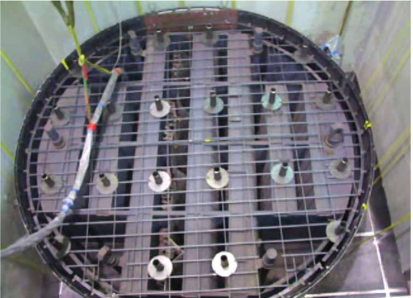
Steam dryer dismantling project—Braun.
